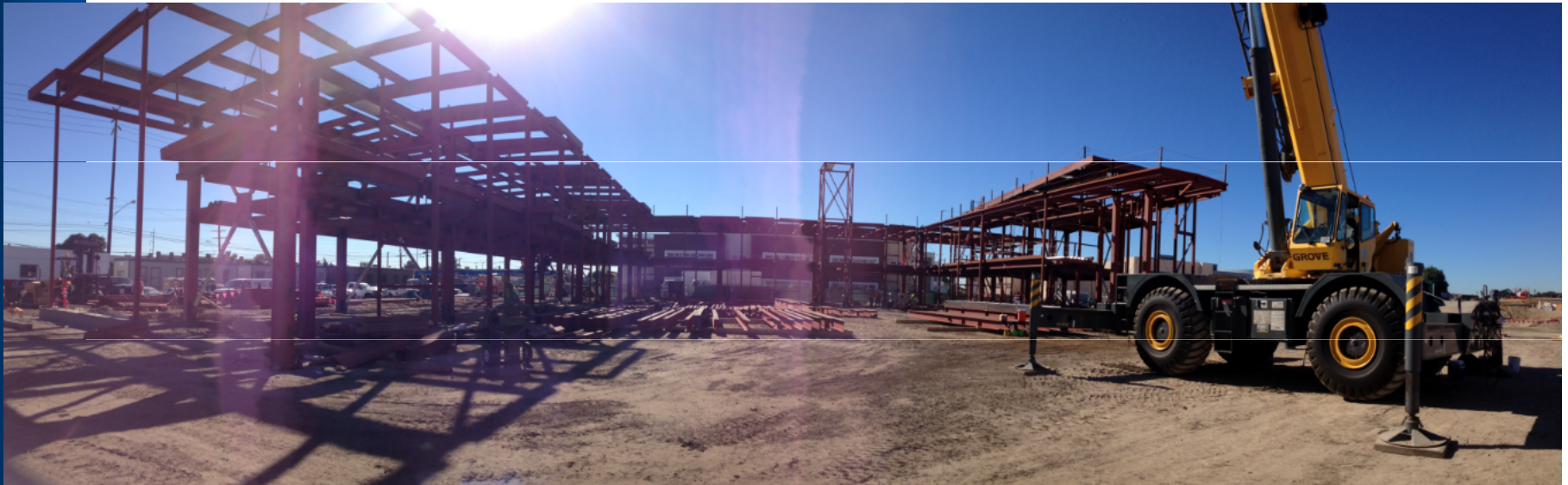
Steel Framing for Engineering Classrooms
